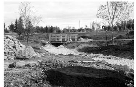
Organic Soil going into a new park in Sherwood Park
