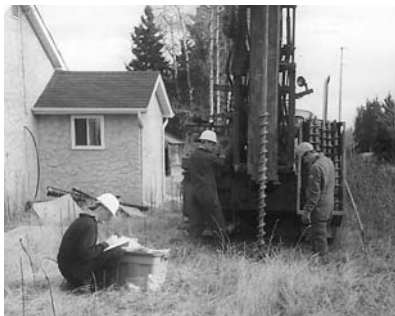
Soil sampling during a Phase II investigation
